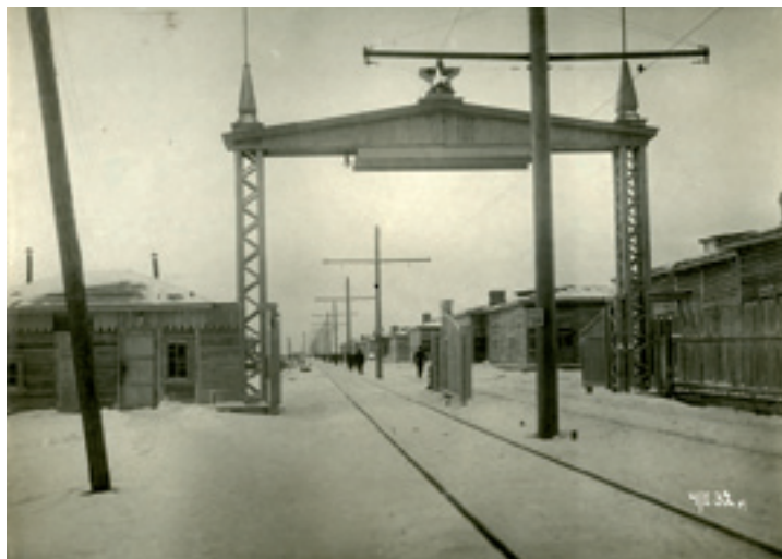
'WORKMEN [']S HOUSES WITH ENTRANCE AND TRAMWAY LINE,' PHOTOGRAPH TAKEN IN AVTOVO ON 4 JANUARY 1932 (IISH)
