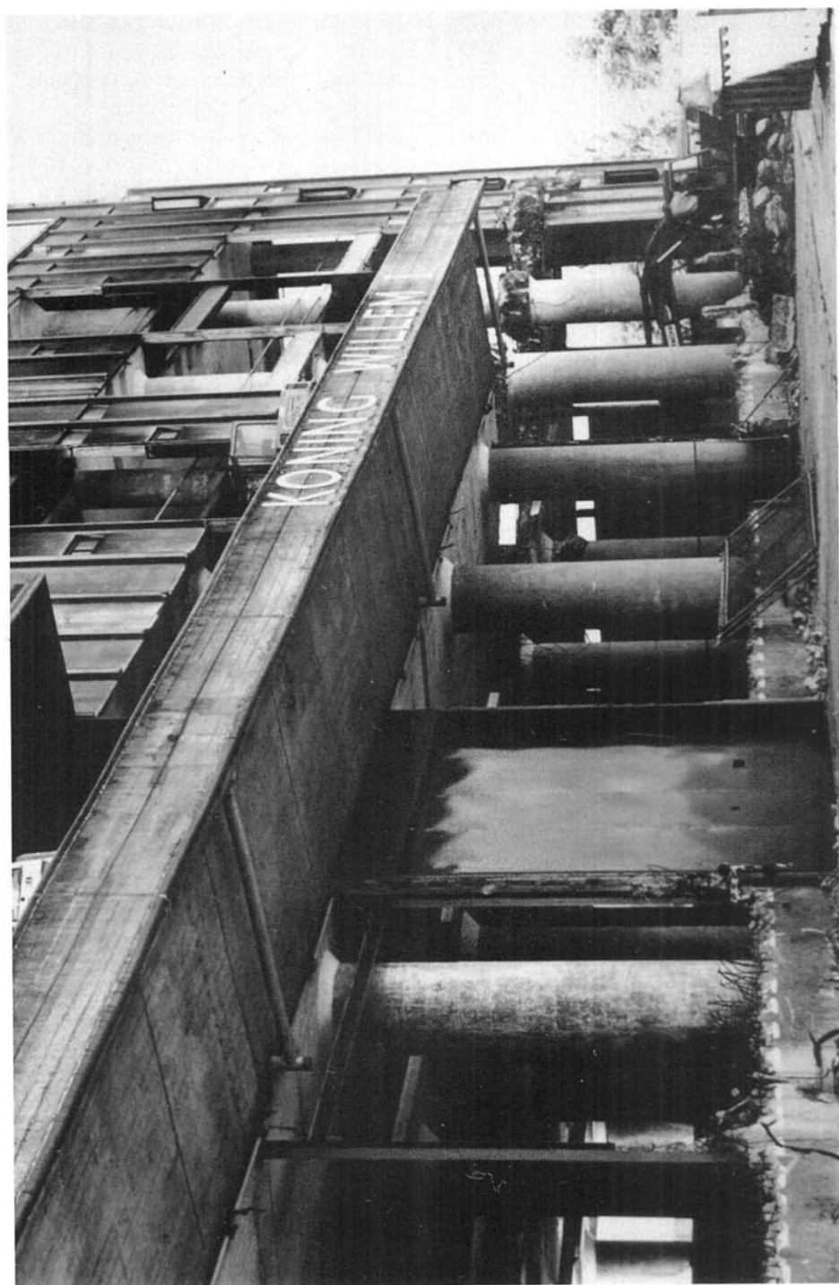
The new building, Cruquiusweg 31, under reconstruction (June 1988). Photo: Eva Strausz.
